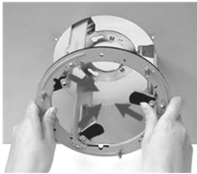
Positioning the flush mount in the ceiling
